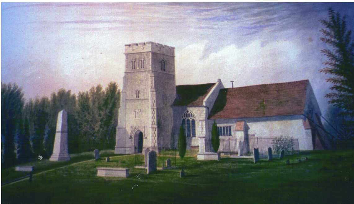
A picture by Henry Davy (1793-1865) showing the former chancel which was demolished in 1872. Note the Clarkson obelisk which was newly erected in 1857 and that the Biddell, Clarkson and Airy railings are already in place. A scattering of headstones and coffin tombs date from the 1830s
